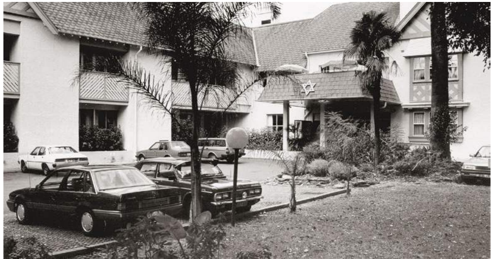
Right: The Hospital following extensive renovations, 1983
